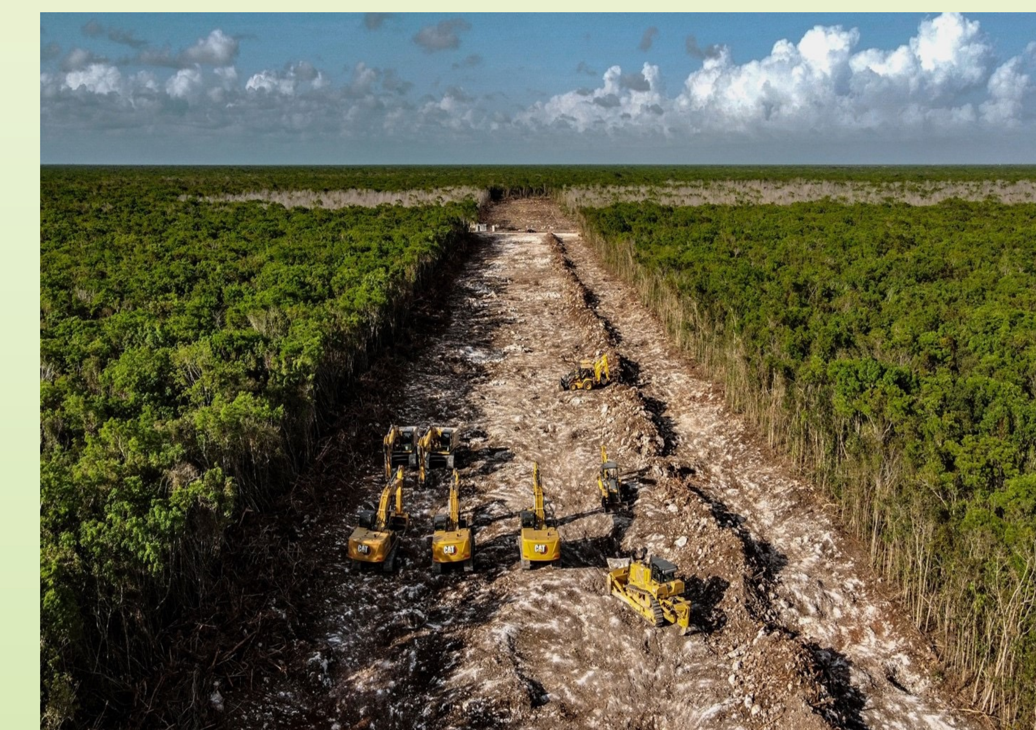
FIGURE 4: Construction of Tren Maya. Photo by Cancun Sun. https://www.nbcnews.com/news/latino/mexico-invokes-powers-build-tourist-train-threat-pre-historic-sites-rcna39102
