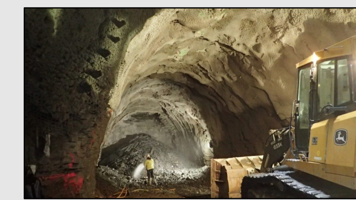
Image Credit: NE Ohio Regional Sewer District
