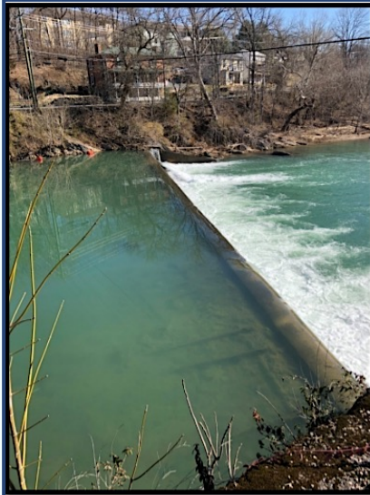
April 2019 (Before Removal)
